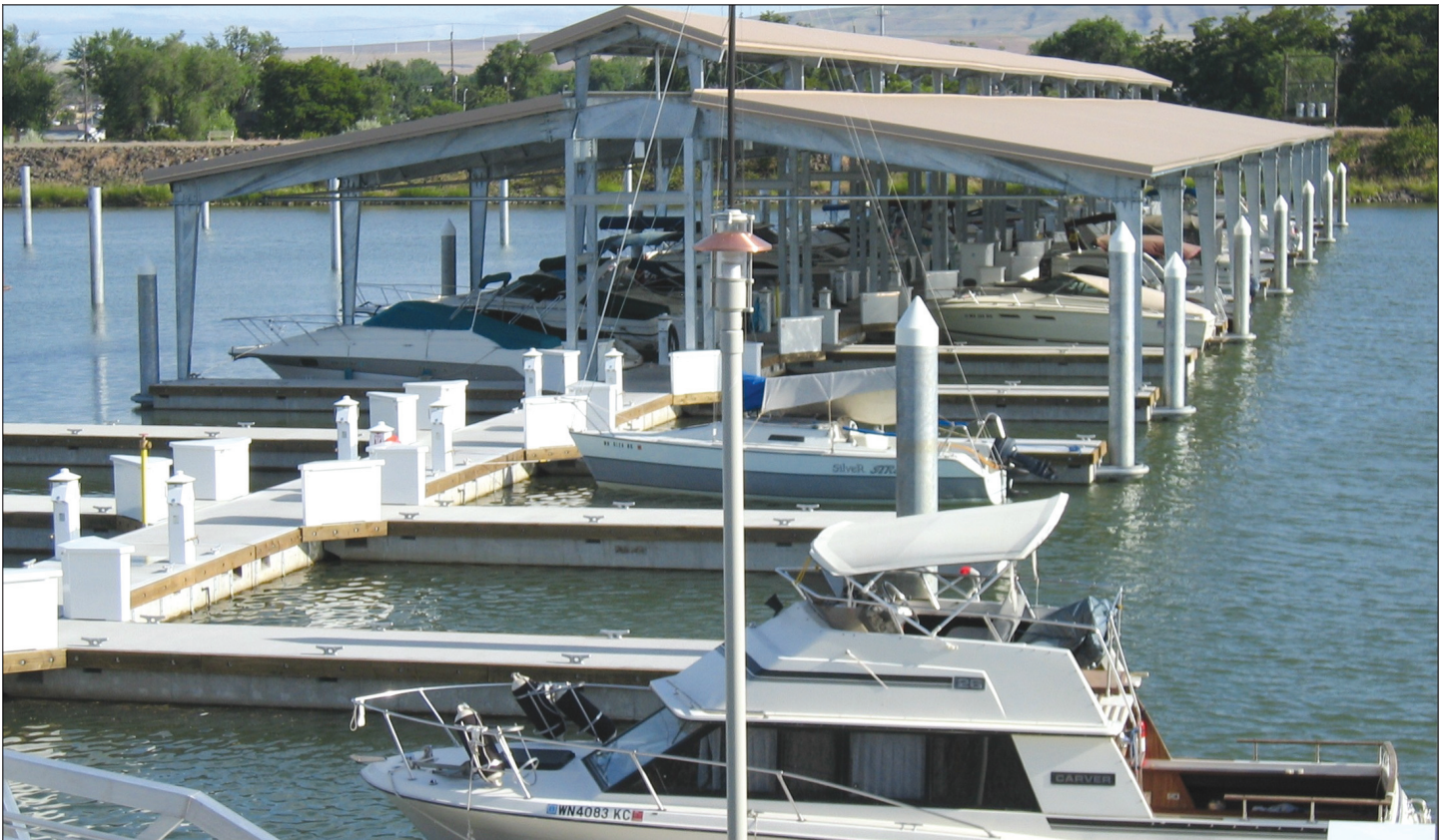
The docks at the new Clover Island Marina in Kennewick have a galvanized structural steel covered moorage.
